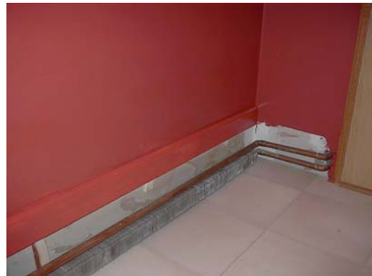
#4 – Paint or finish off the spacer board in the desired color.
