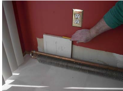
#2 – Create a template to mark where the top rail of the new Radiant Wraps panel will sit against wall (height is determined by the size option selected).
