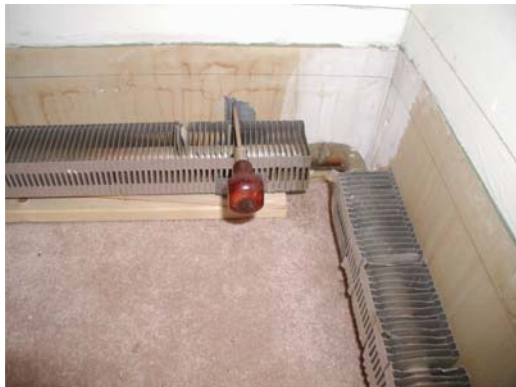
#3 – Slide support bracket into place and prepare starter hole for screw mounting.
