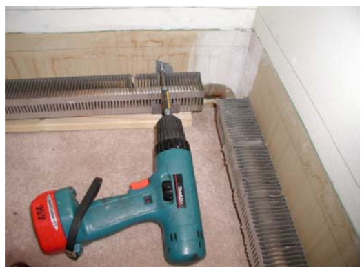
#4 – Level off heating element and install screw to anchor support bracket to wall.
