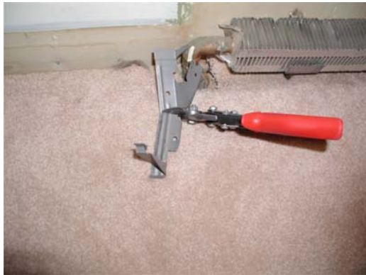
#1 – Refer to Removing Existing Back Panels & Support Brackets page for preparation. Snip off support brackets at appropriate height as determined by Radiant Wraps.
