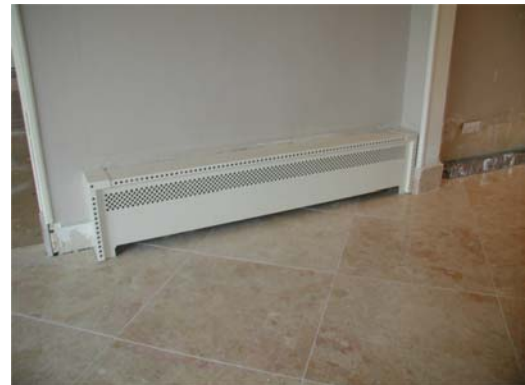
#6 – Slide back flange of new panel down into mounting brackets.
