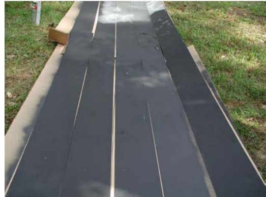
#2 – A 6-inch high coil of tin roof flashing should be rolled out and cut to cover the wall area. Paint the silver flashing with a flat black paint (Rustoleum).
