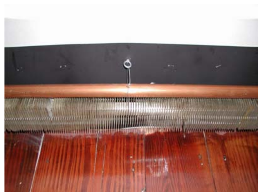
#4 – A hook & eye screw, & wire support should be installed at 6" off the floor every 3 to 4 feet. (See Hook & Eye Support for detail).
