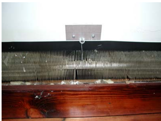
#5 – The mounting brackets are installed (see Mounting Bracket Installation page for more detail).
