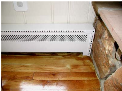
#5 – Install new panel and end cap.
