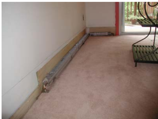
#5 – Once back panel has been detached from wall, slide it up and out.
