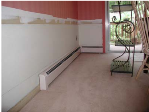
#1 – Remove all existing snap on or slide on components to prepare enclosure for removal.
