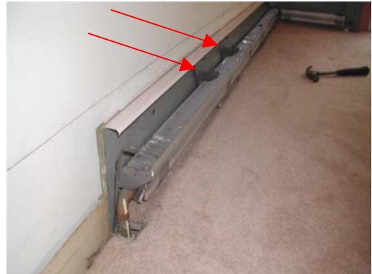
#2 – Use hammer to loosen support brackets and slide them horizontally to the closest opening (they will be re-used).
