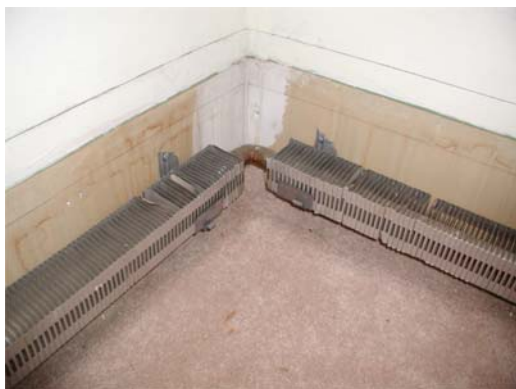
#5 – This photo shows support brackets re-attached.
