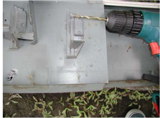
#2 – In the event that the pre-drilled holes have been snipped off, re-drill a hole for re-mounting the support bracket to the wall.
