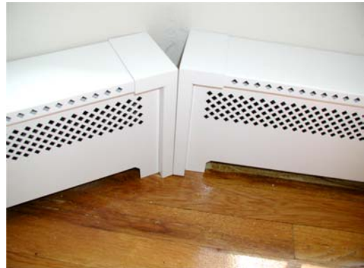
#4 – The left open end cap will be installed tight to the right open end cap.
