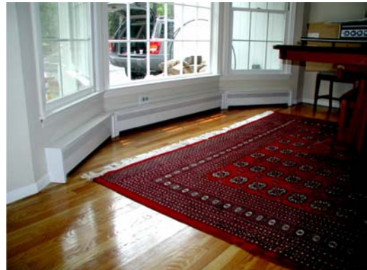
#6 – A finished non-90 degree corner. Please allow 30-days for Radiant Wraps to fabricate the custom top rail wedge piece.
