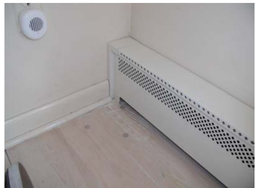
#6 – Slide new end cap down into place.
