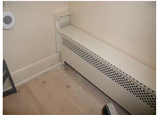
#2 – Use straight edge to mark notch line down across base molding.
